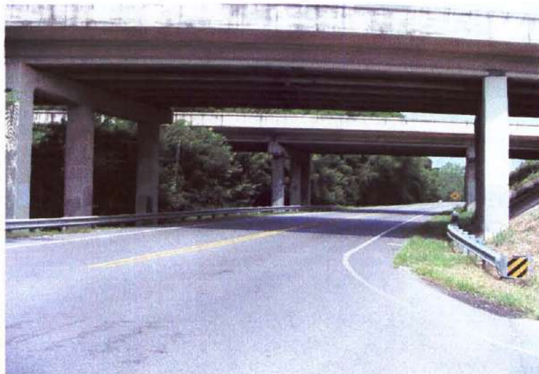
Looking Ahead on Route (94-106-5.88)
