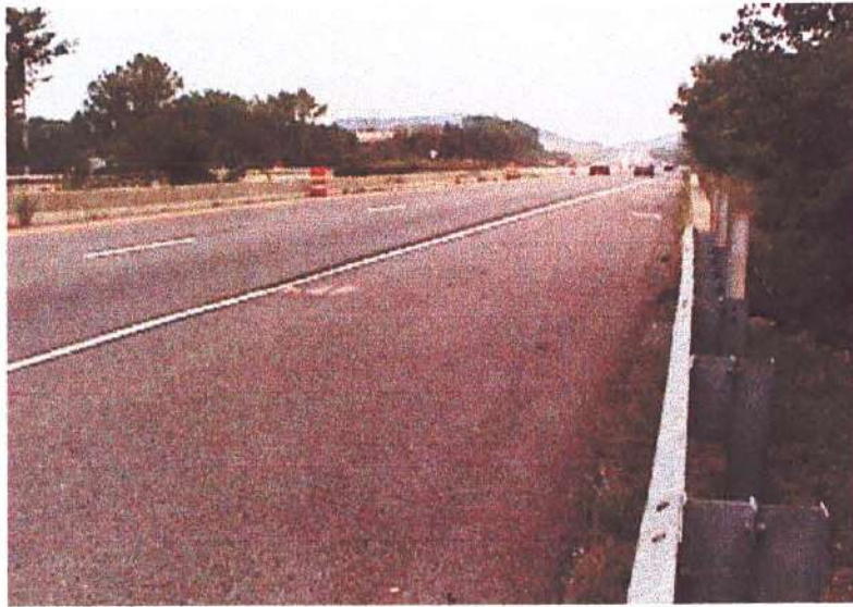
ACROSS TOP OF DECK
