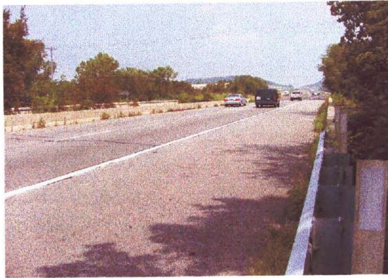
ACROSS TOP OF DECK
