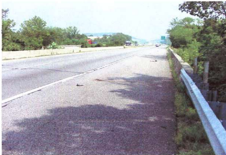
Across Top of Deck
